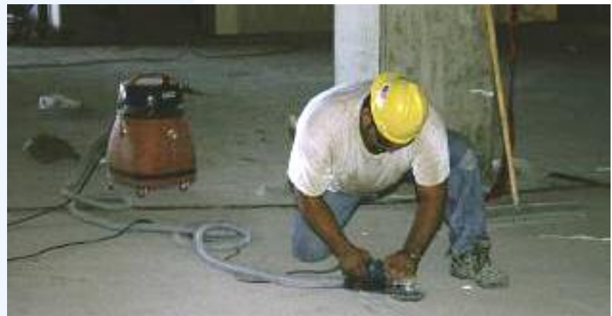
Grinding, using a vacuum dust collector
