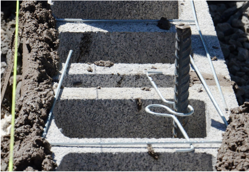
This photo shows splicing before full mortar coverage was applied.
