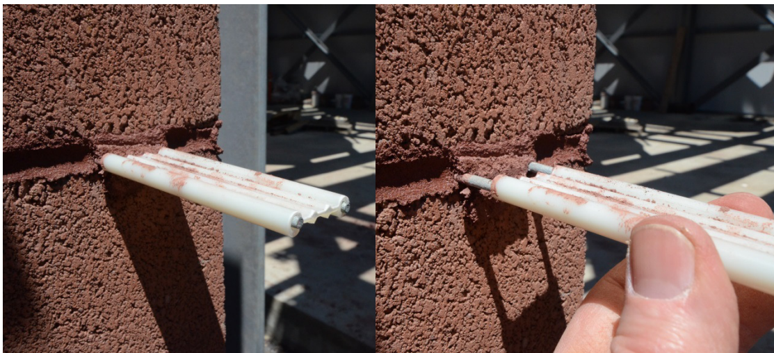
Typical slip anchor
