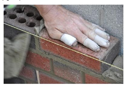
Figure 2 – "Solid" brick unit laid in a full bed joint with a full head (end) joint
