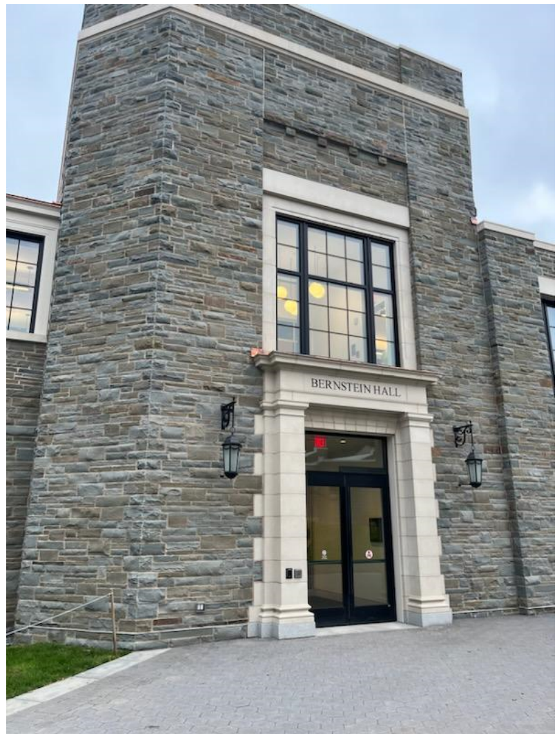
Front Entrance showing special corbel stone units above window
