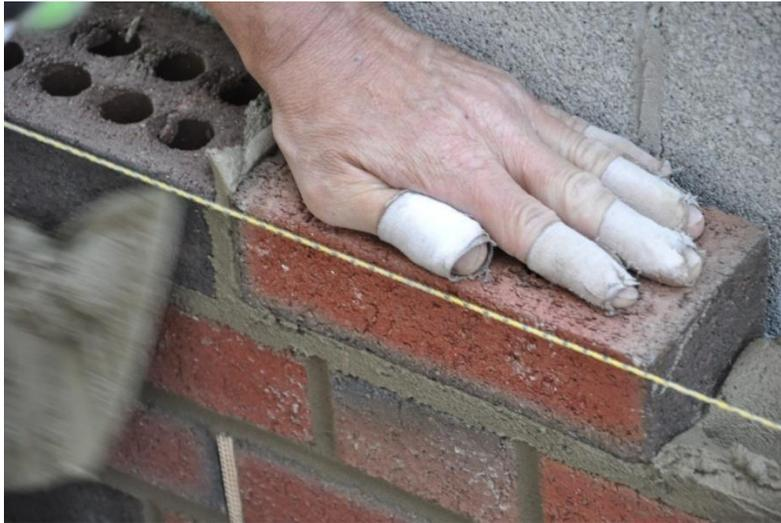
Figure 2 – “Solid” brick unit laid in a full bed joint with a full head (end) joint
