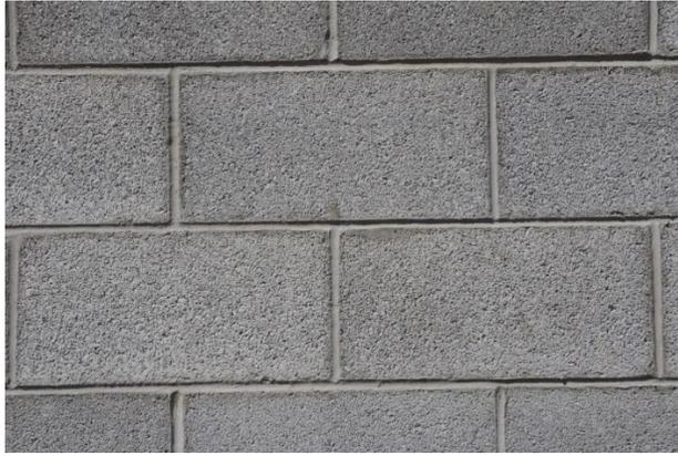
Figure 6 – Sound bed and end joints in “hollow” CMU
