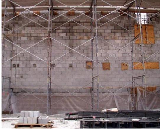
Figure 4 – Grout cleanouts in the second pour
