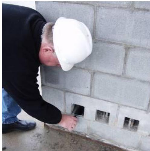
Figure 1 – Grout cleanout
